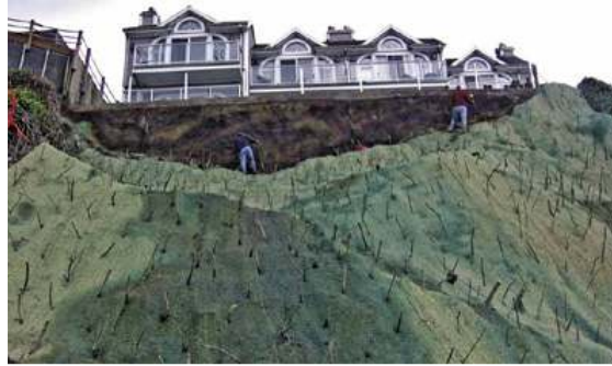
A remediation project of severe soil erosion on the Oregon Coast.
